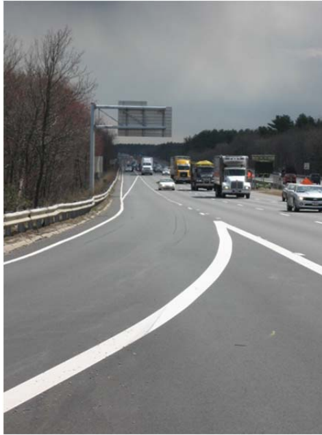
Figure 70. Photo. Off-ramp striping, I-93.
