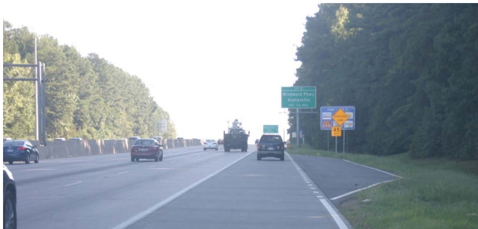
Figure 36. Photo. Emergency Turnout, Georgia.
