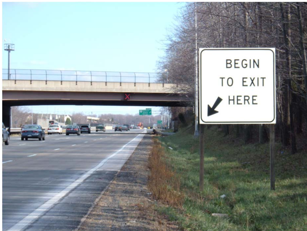
Figure 63. Photo. Static signage denoting permitted use of shoulder to exit during non-operational hours of shoulder use, I-66 mainline.
