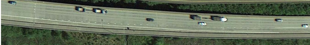
Figure 67. Photo. Edge line markings at the start of part-time shoulder use segment, US 2. (Source: Google Earth)
