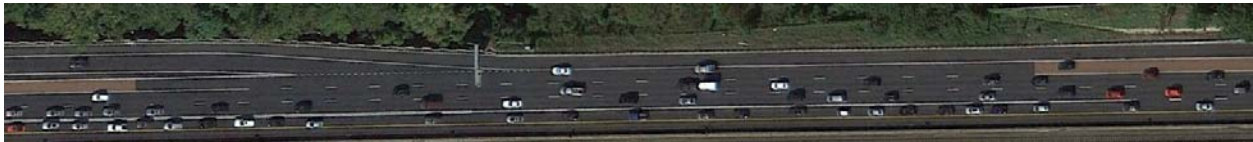
Figure 71. Photo. Off-ramp striping, I-66.
