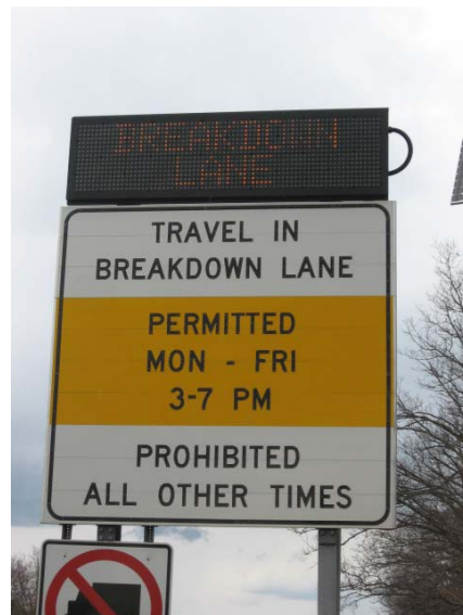
Figure 56. Photo. Dynamic sign signifying the shoulder is closed to traffic, I-95 breakdown lanes. (Source: Massachusetts Department of Transportation)
