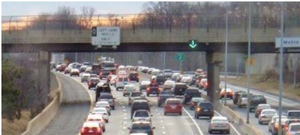
Figure 5. Photo. Previous Static Part-time shoulder use on I-66 in Northern Virginia (Source: Virginia Department of Transportation)
