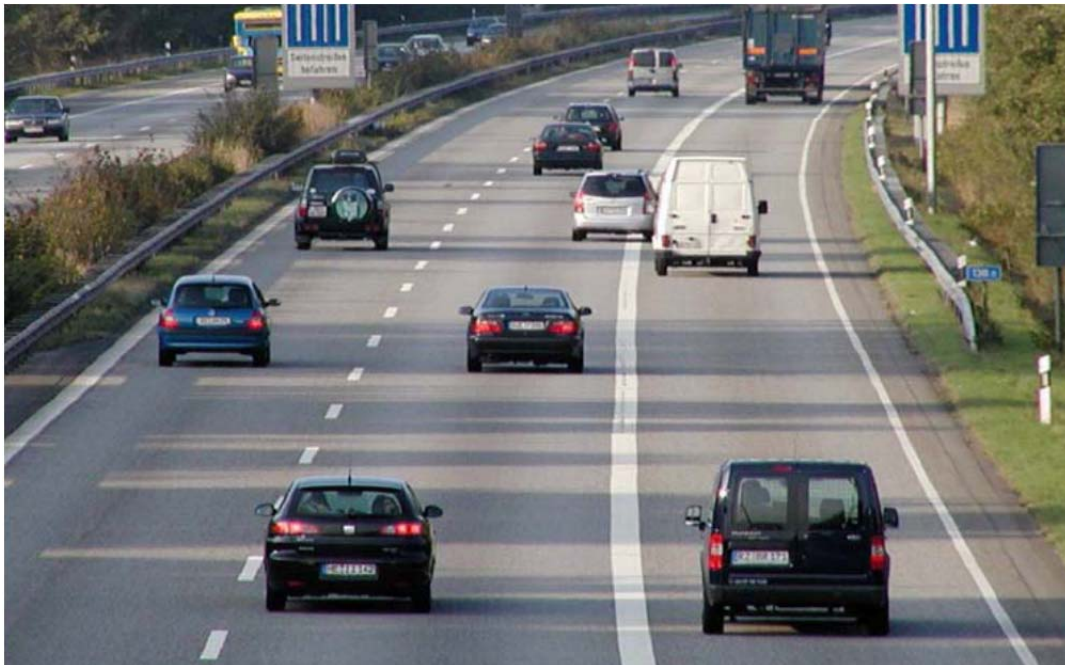
Figure 7. Photo. Part-time shoulder use in Germany.
