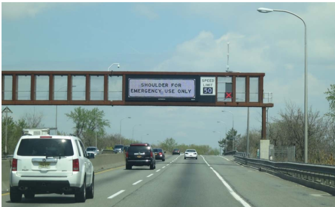
Figure 60. Photo. Dynamic Lane Control Sign on Gantry, New Jersey Turnpike Newark Bay Extension.
