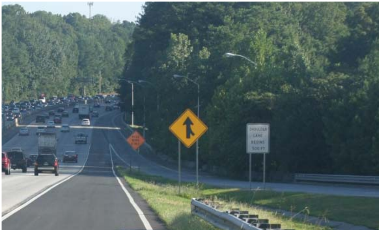
Figure 50. Photo. Regulatory sign on on-ramp, GA 400 (Source: Georgia Department of Transportation)
